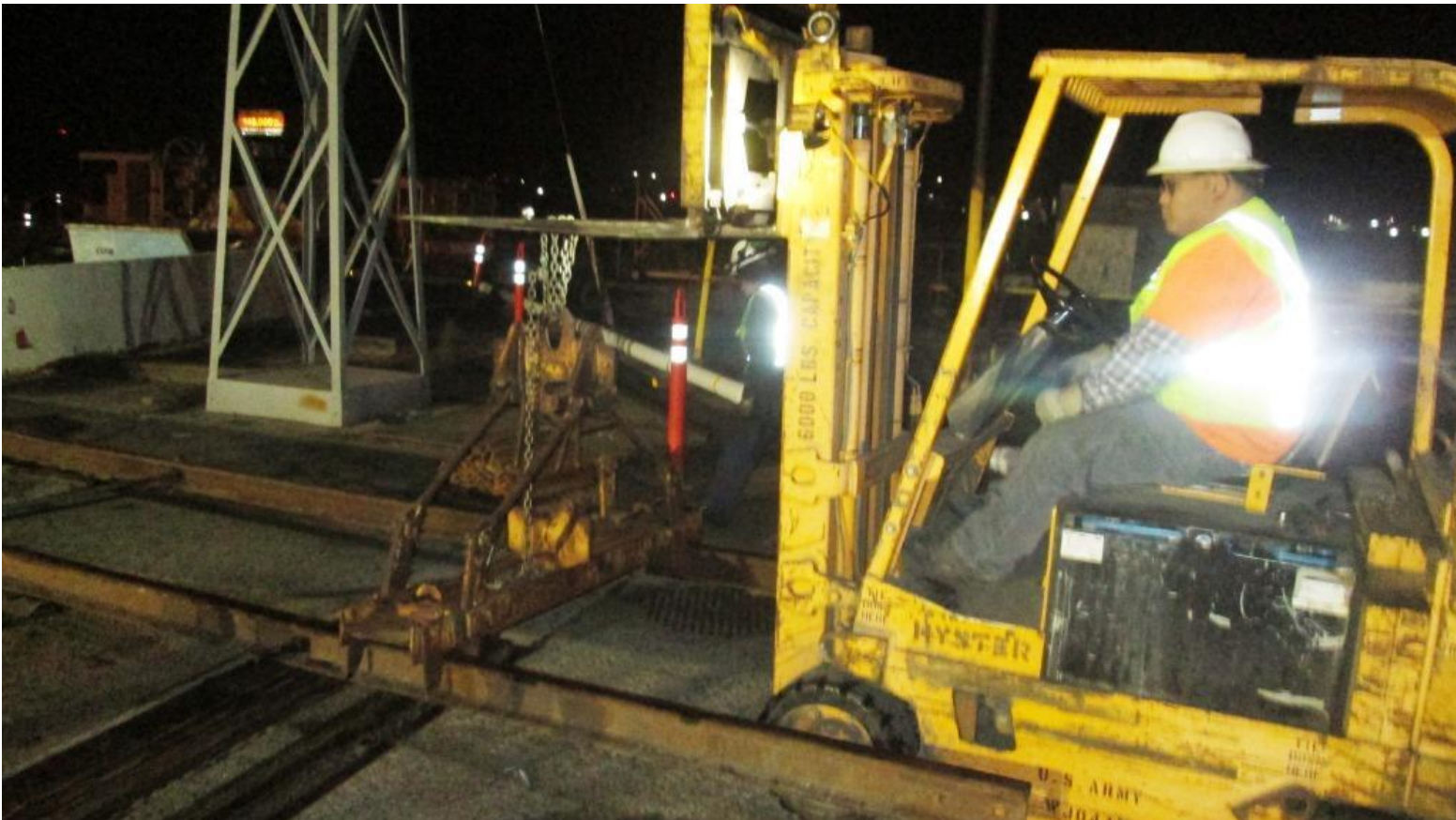
Anthony uses the forklift to attach the panel-track lifter to the section of temporary track being moved out on the transfer table runway
