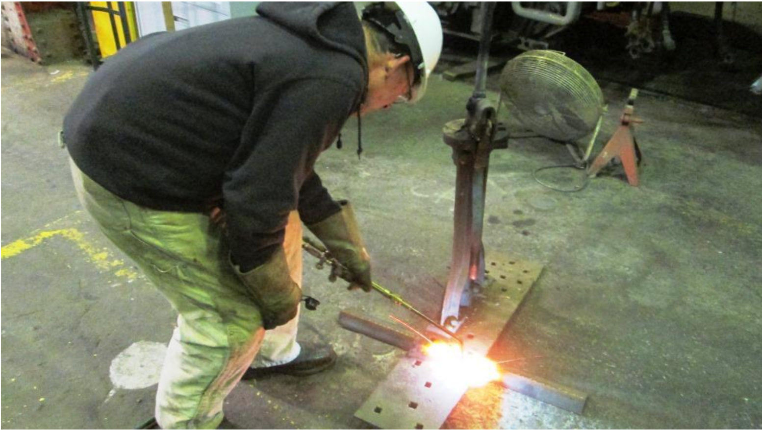
Cliff heats the base of the replacement switch-stand for Switch 2 in order to bend it straight
