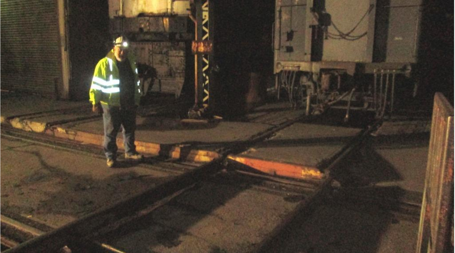
Frank guides the lining of the temporary track to the South Firing-Line track
