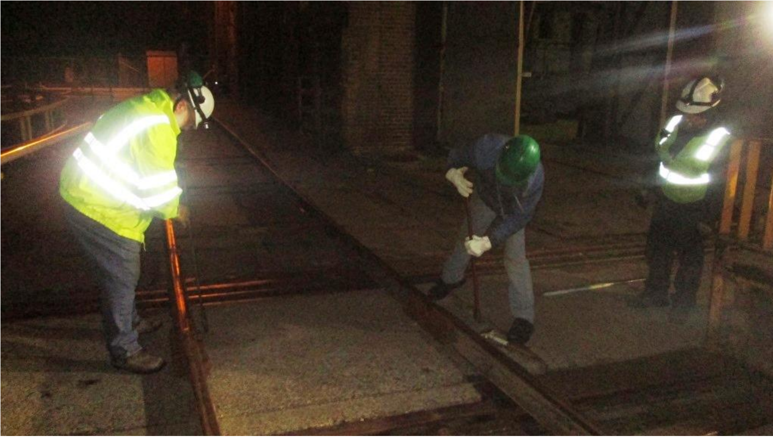
After attaching joint-bars, Frank and Paul tighten down the bolts
