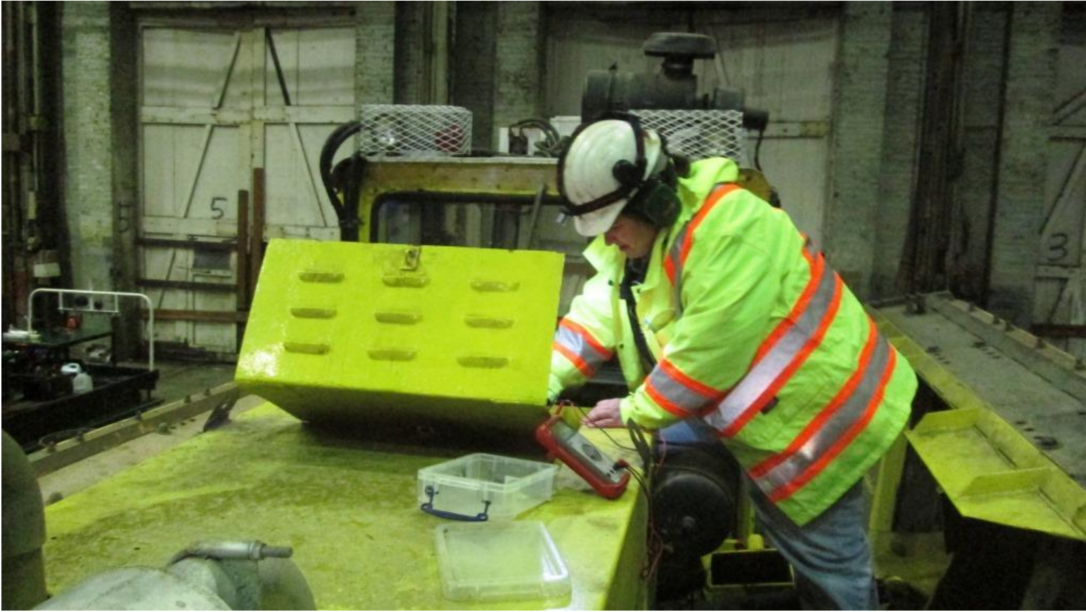
Heather hunting down the electrical “parasite” on the ballast regulator
