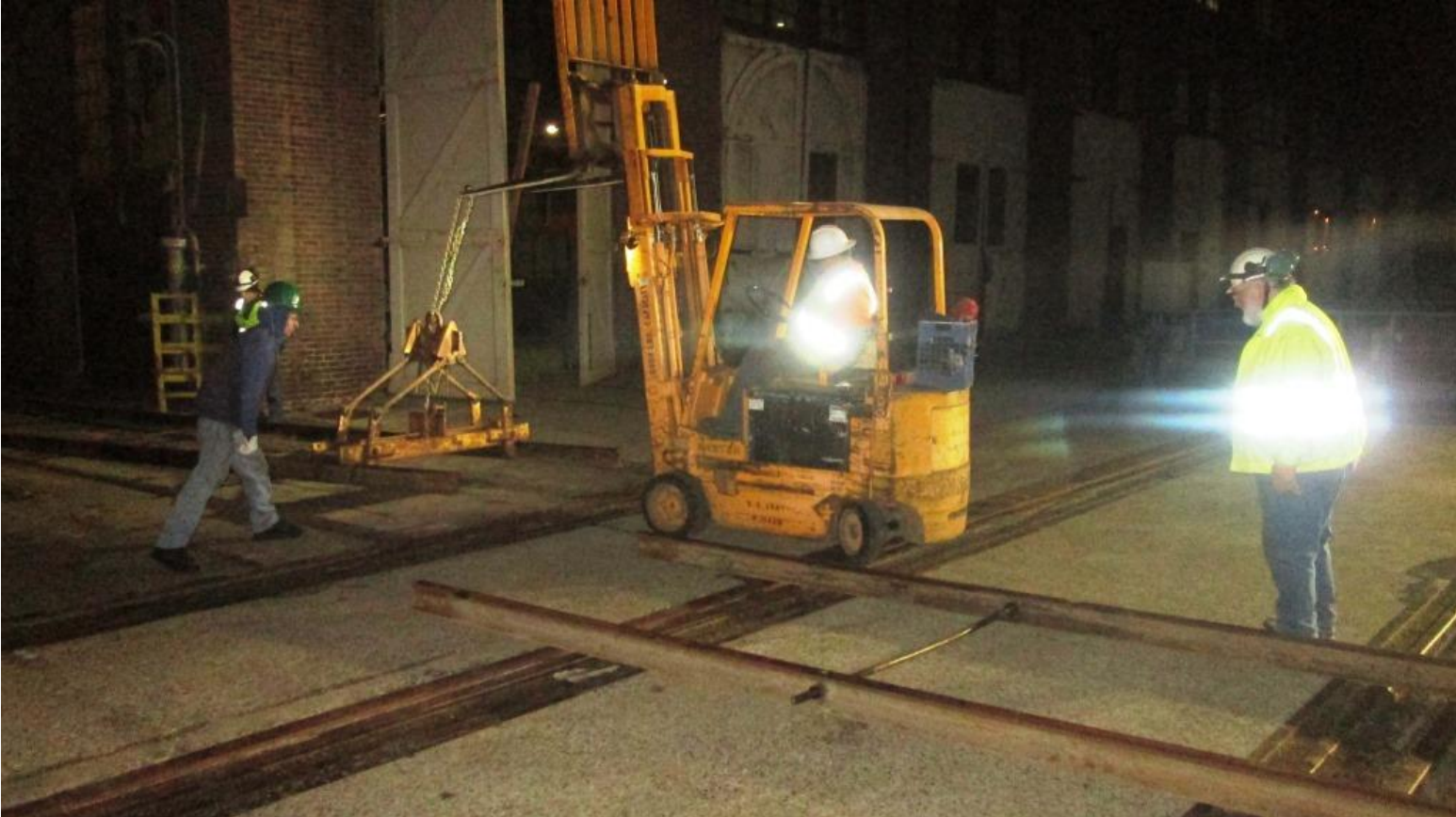
The second section is dragged over to meet up with the first section
