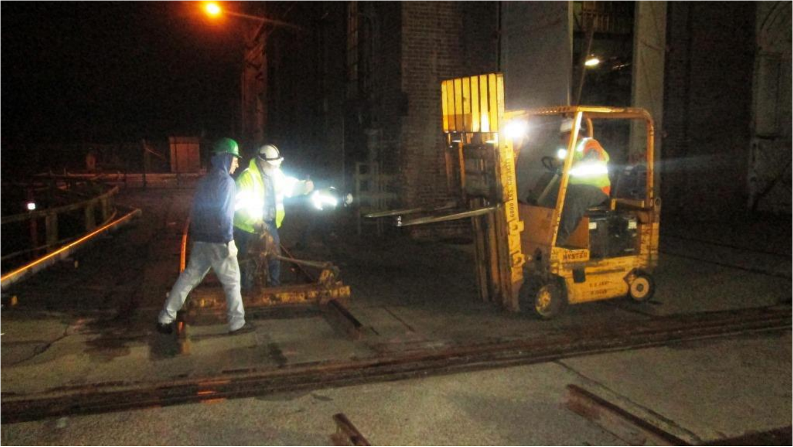
With the first section of track lined-up, Paul and Frank guide Anthony in grabbing the panel-track lifter to move the second section
