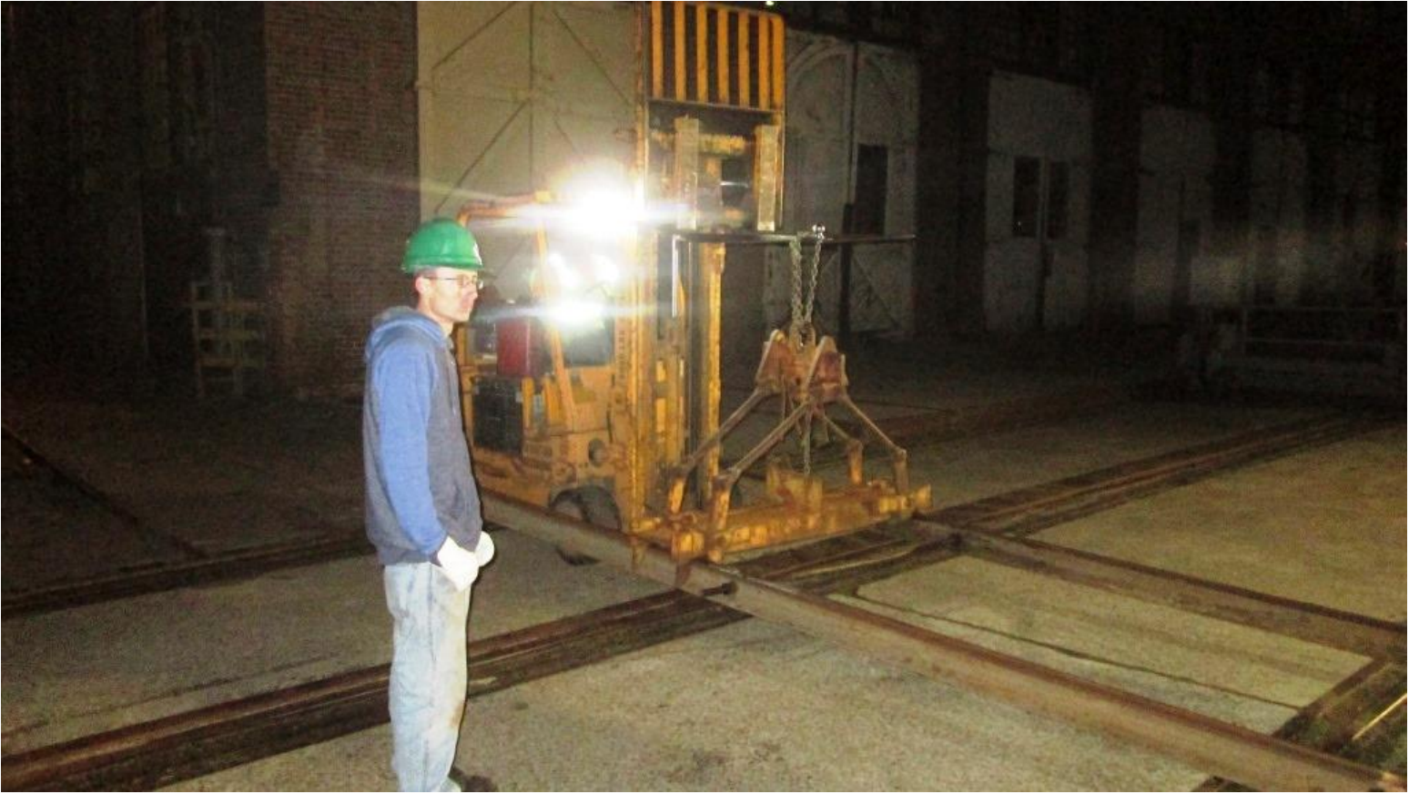
Paul stands by to relay signals as Anthony on the forklift lifts the rails
